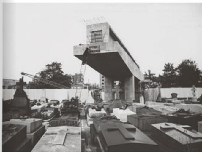
The Périphérique in construction over the Batignolles Cemetery.
